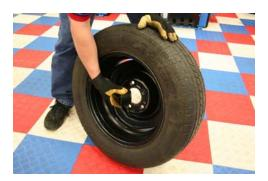
**STEP 3:** Place the cone on the shaft.
